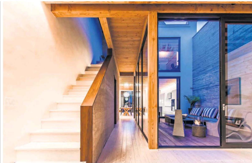
In Sabine Karsenti’s custom-built home in Montreal, walls are made from a composite of hemp, crushed limestone and sand. ALEXANDRE PARENT/STUDIO POINT DEVUE
