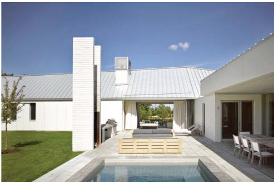
The choice of low-maintenance construction materials such as cement-board siding, aluminium windows and a steel roof on the exterior minimises future repair and ensures that the building would age gracefully.
